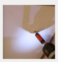
**5.** While holding the boards in position use suitable length drywall screws to fix the board into the timber joist. Screws should go into the joist at least 35mm. We recommend a screw every 200 - 300mm on each joist. The screw head should be flush with the board when screwed into place.
