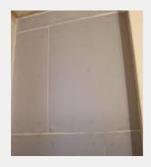
7. Start the second row from where the first ended to give the boards a staggered joint. Follow the same procedure until the ceiling is completed. Ensuring the first board is flush and square will make the rest of the installation easier.
