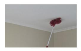
**2.** Make sure the ceiling is flat, clean and that all dust is wiped away. Fill any gaps in existing plasterboard with acoustic sealant.
