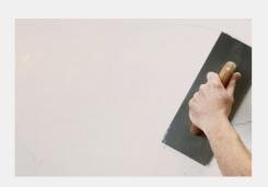
9. The SoundBoard 4 is then ready for standard plasterboard finishing.A plaster skim finish is most common but heavy duty backing paper can also be used.
